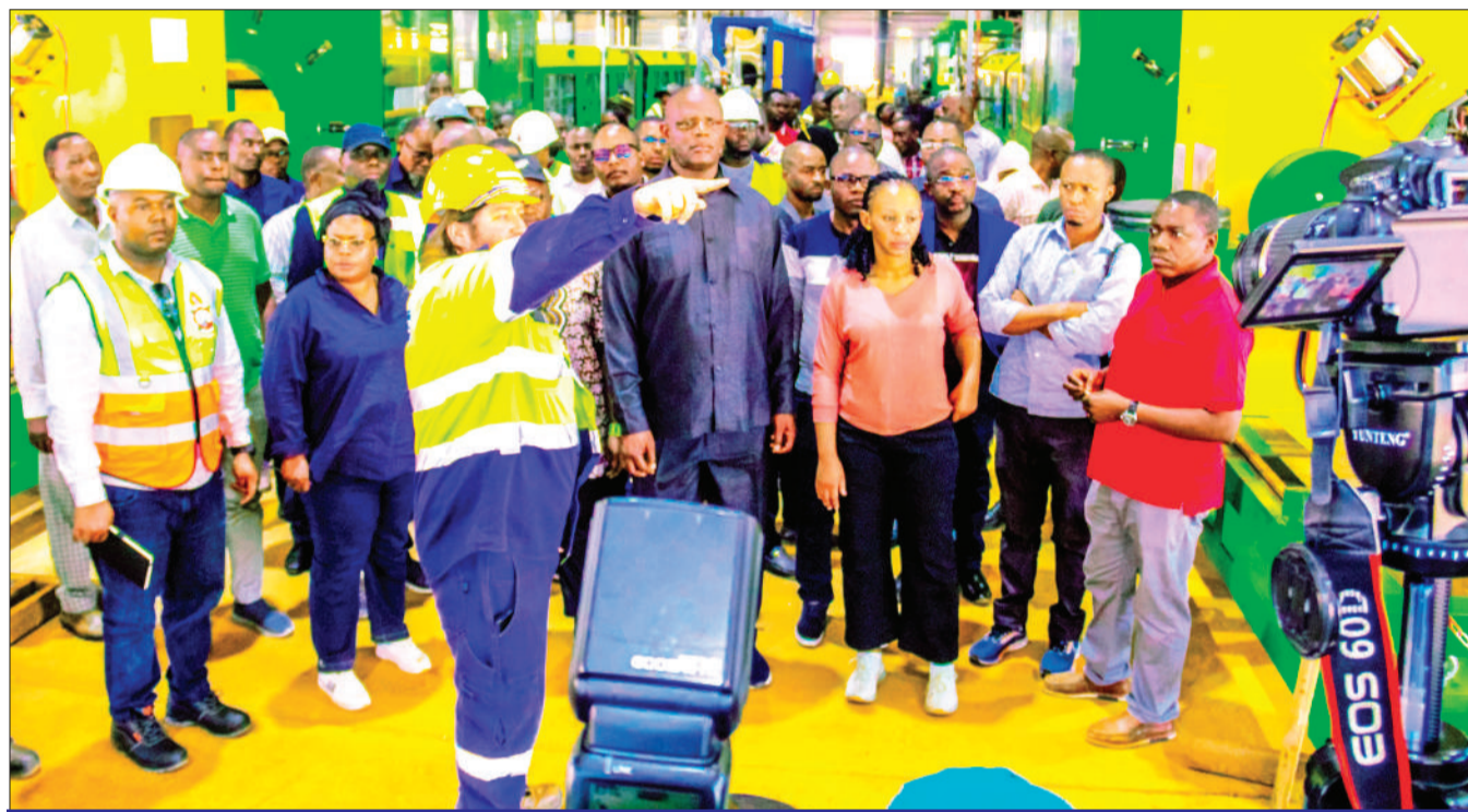
Guillaume Mallevey (in yellow helmet), an oil heating systems and factory construction manager with the East African Crude Oil Pipeline (EACOP), briefs members of the Parliamentary Standing Committee on Public Accounts who visited the project's site at Sojo village in Nzega District, Tabora Region, on Tuesday. Photo: Correspondent Marco Maduhu
