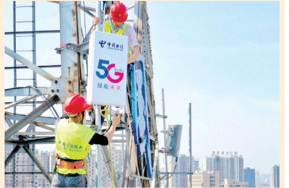
Employees with China Telecom's Lu'an branch install and test a 5G base station in downtown Lu'an, east China's Anhui province, May 4, 2020. (Photo by Tian Kaipeng/People's Daily Online)
