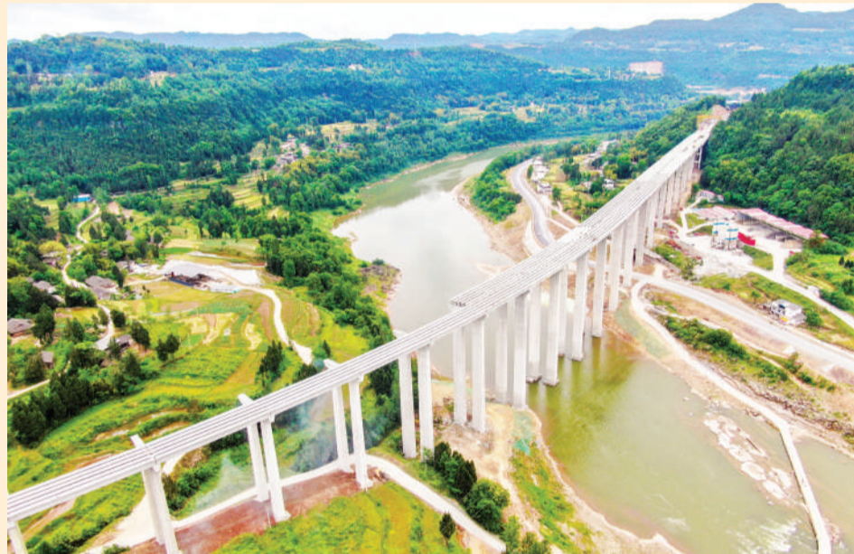
Photo taken on May 8 shows an aerial view of the extra-large bridge over Tongjiang river in Bazhong, southwest China's Sichuan province. The bridge, which is a part of an expressway connecting Bazhong and Wanyuan, opened to traffic on May 5. (Photo by Cheng Cong/People's Daily Online)
