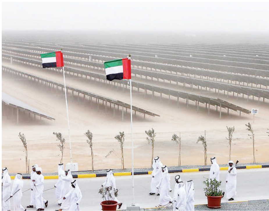
The Mohammed bin Rashid Al Maktoum Solar Park is set to have a capacity of 5,000 megawatts by 2030.
