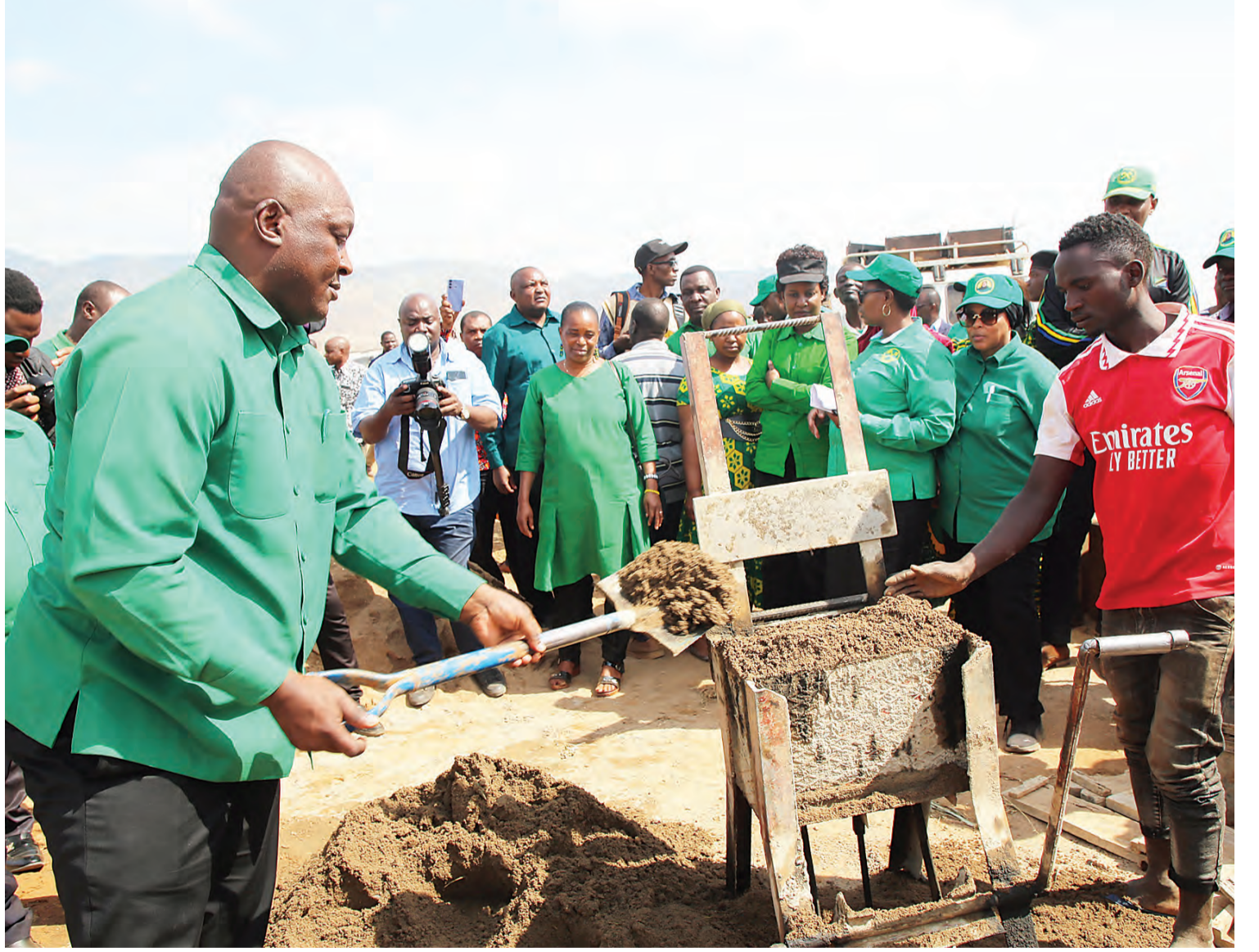
CCM Secretary General Daniel Chongolo lends a hand in the making of bricks for use in construction work at Kingiti Ward Secondary School in Mpwapwa District, Dodoma Region, yesterday while on a visit to Kibakwe constituency. Photo: Correspondent Ibrahim Joseph
