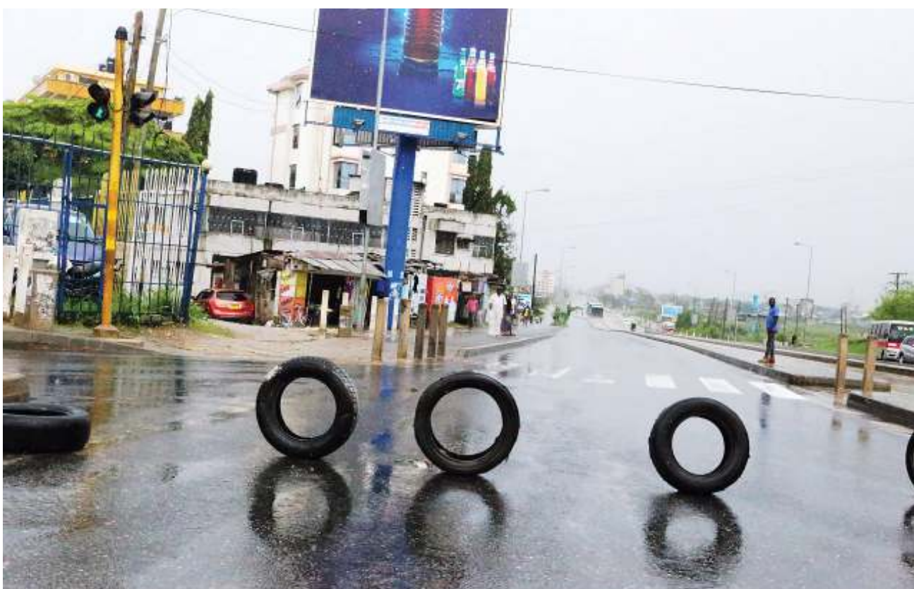
Used tyres installed by traffic police officers along the Fire section of Morogoro Road in an effort to keep motorists away following floods in the Jangwani Valley.
