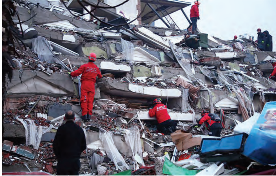
Rescuers search for survivors on the rubble of a building destroyed in a powerful earthquake in Kahramanmaraş, Türkiye, on Feb. 7, 2023. (Xinhua/Li Zhenbei)
