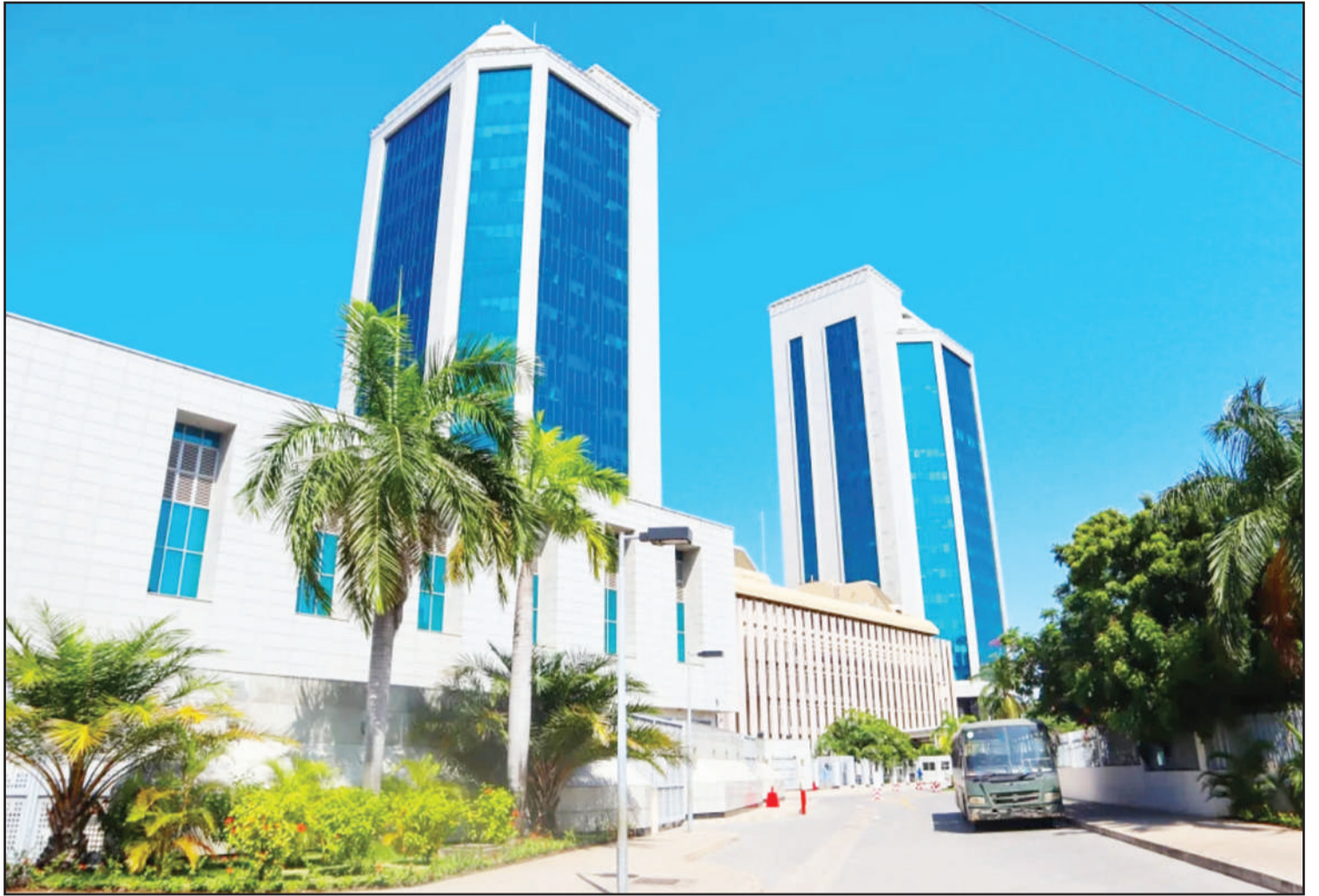
Side view of the central bank's twin towers in Dar es Salaam. File Photo.
