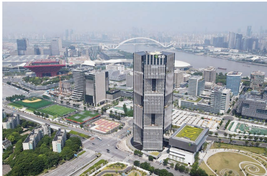
Aerial photo taken on June 17, 2022 shows the headquarters building of the New Development Bank (NDB), also known as the BRICS bank, in east China's Shanghai. Photo: Xinhua
