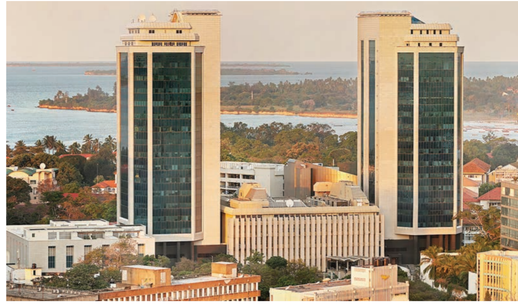
BoT headquarters in Dar es Salaam
