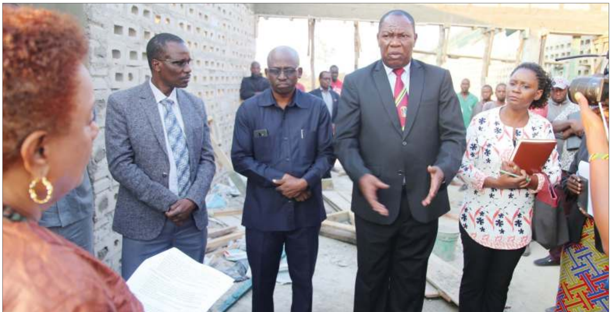
Tabora regional commissioner Aggrey Mwanri (2nd R) stresses a point during his visit to the construction site of infrastructures in Sikonge district hospital yesterday. Photo: Daud Tiganya
