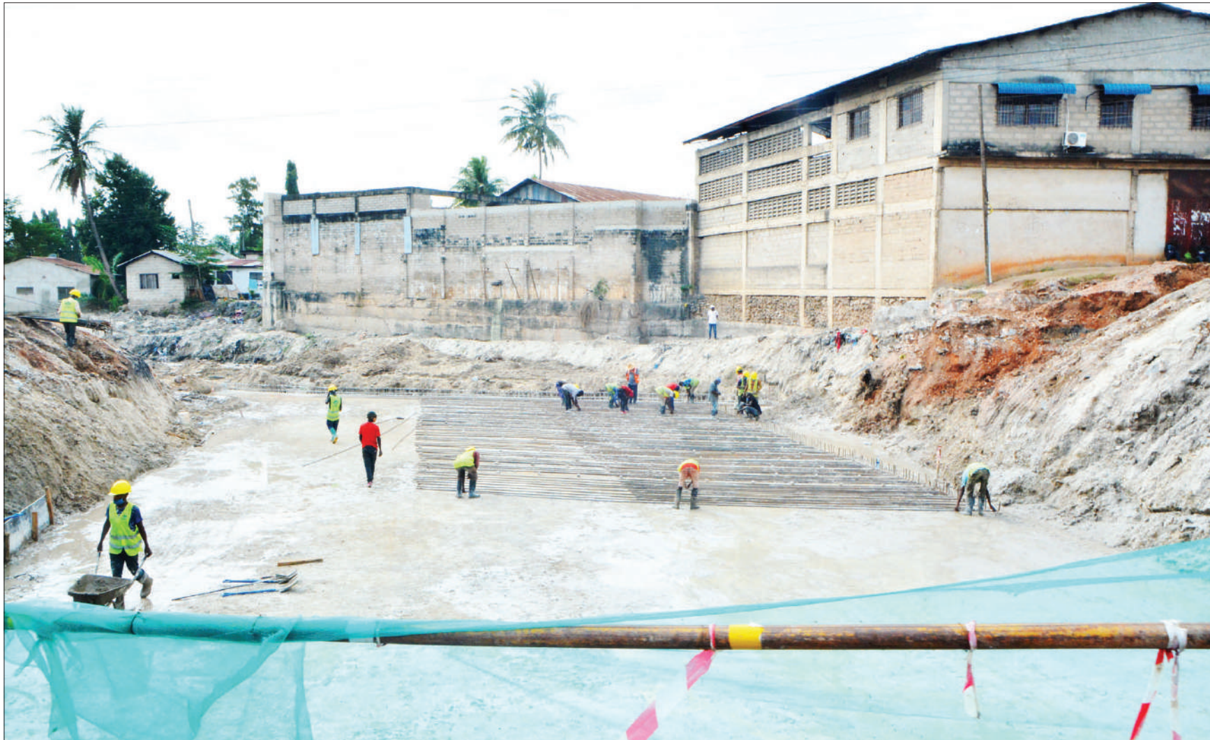
Efforts to reinforce the Ng'ombe River bed and banks as part of a strategy to mitigate the impact of flooding are making steady progress, as witnessed close to a stretch of Dar es Salaam's Shekilango Road yesterday. Photo: Correspondent Miraji Msala
