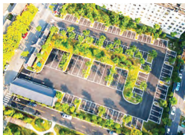
Photo taken on Aug. 20, 2020 shows a "sponge parking lot" in Rugao, east China's Jiangsu province. (File photo)
