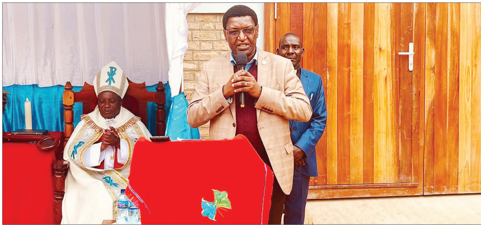
Joseph Chilambo, a representative of the TIB Bank managing director, pictured earlier this week speaking during the laying of the foundation stone for Ijangara mini-hydropower project, which is being executed by the Evangelical Lutheran Church in Tanzania (ELCT) through Lutheran DKK Energy Company. The firm is based at Msiwiwe village in Makete District, Njombe Region, while the project is being implemented thanks to funding to the tune of USD 400000 as a TIB loan, a Rural Energy Agency subsidy and support by various other stakeholders. Left is ELCT Presiding Bishop Dr Fredrick Onael Shoo. Photo: Guardian Correspondent
