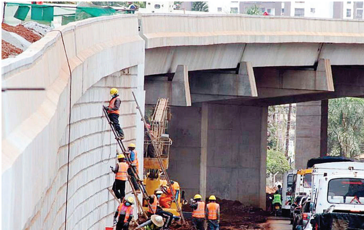
Ongoing construction of the Nairobi Expressway Uhuru Highway.
