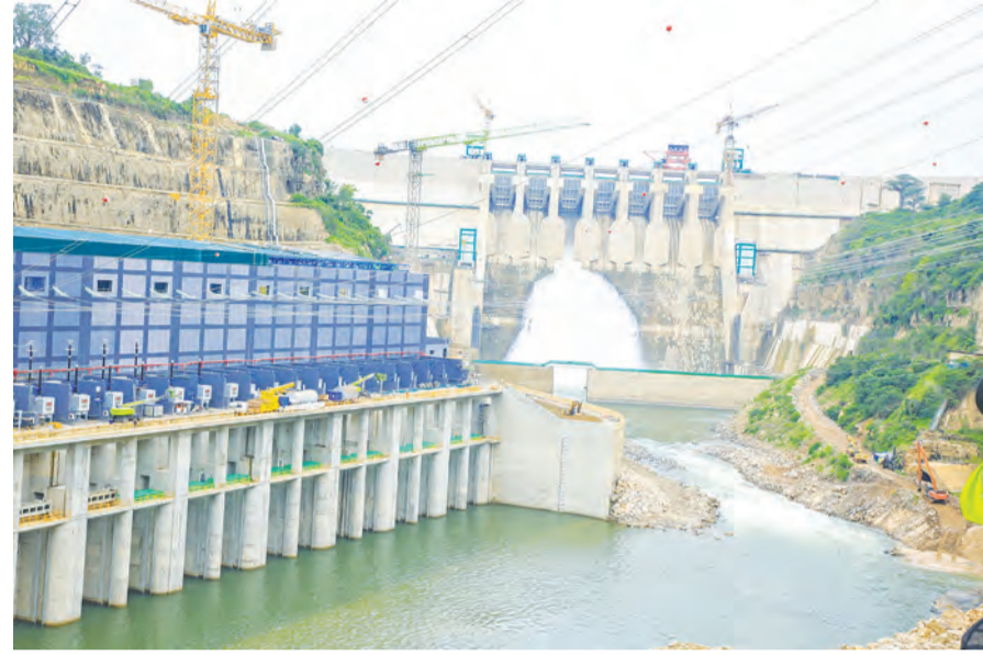
The operationalization of one turbine at Julius Nyerere Hydro-Power Plant has helped to increase the generation of electricity. File Photo
