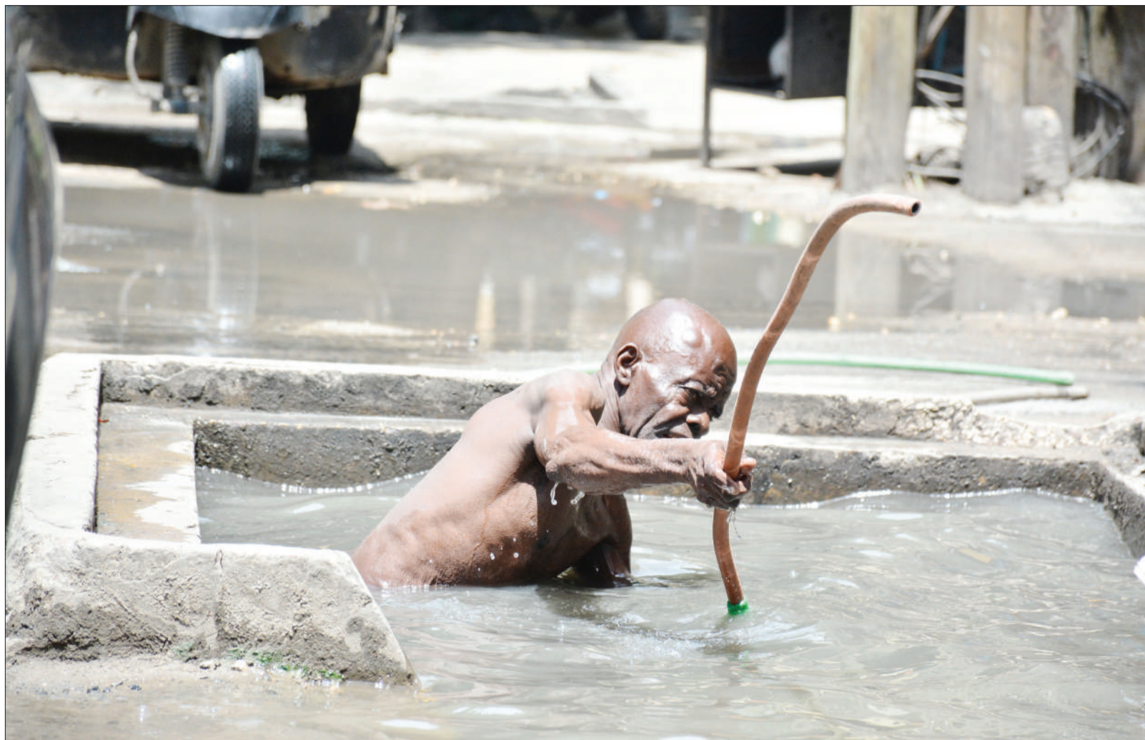
Dar es Salaam resident clears a storm water drain which got clogged with sand, mud and leaves along Udoe/Livingstone Streets in Dar es Salaam yesterday. Photo: Correspondent Miraji Msala
