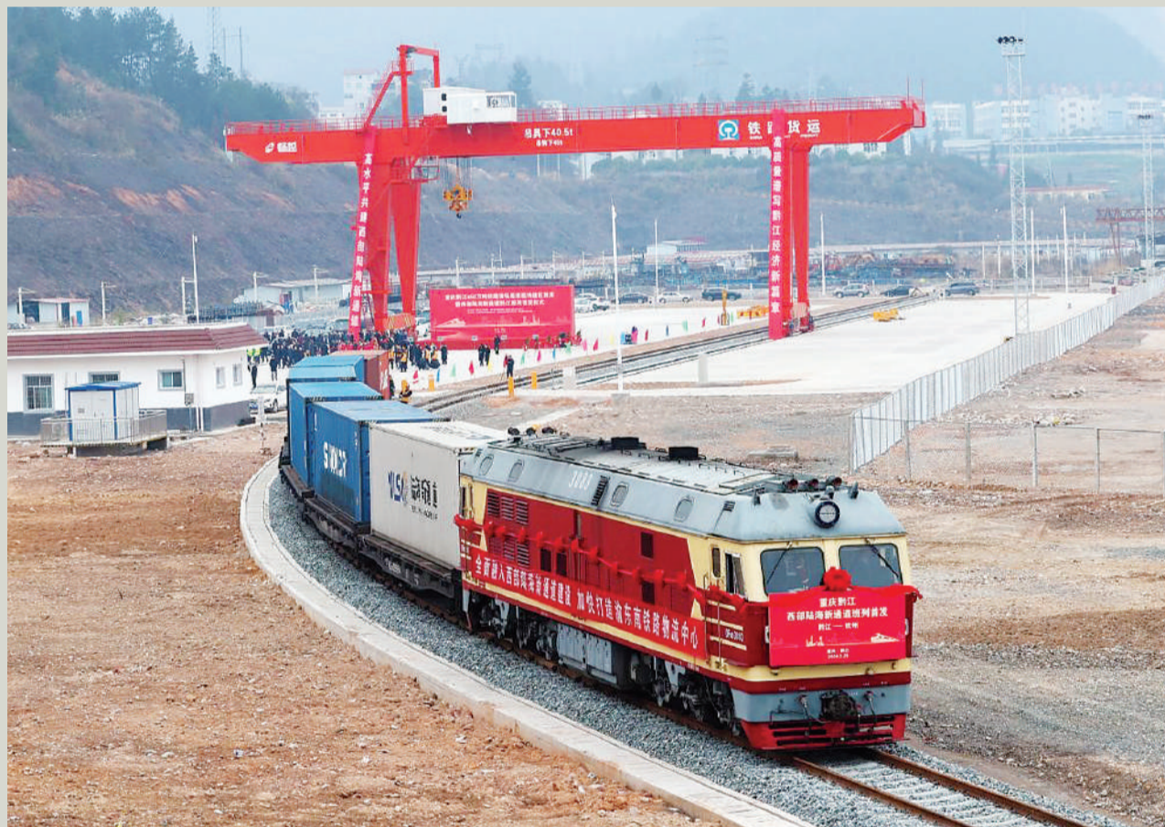
A container yard with a capacity of 4.5 million tons was put into operation at the Qianjiang Railway Station along the Chongqing-Huaihua Railway on Feb. 29, 2024. Photo shows the first train departing from the Qianjiang Railway Station to run along the New International Land-Sea Trade Corridor (ILSTC). (Photo: Yang Min/People's Daily Online)
