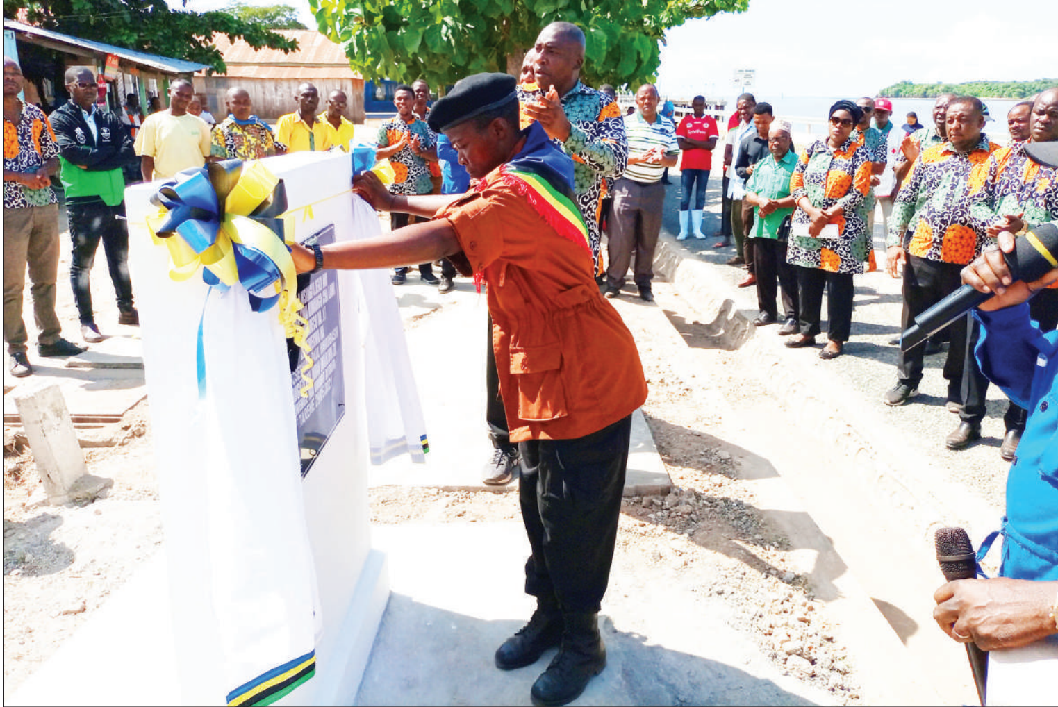
Uhuru Torch race leader Josephine Paul lays a foundation stone for the construction of Pwani-Pangani Road in Tanga Region over the weekend. Photo: Correspondent Steve John
