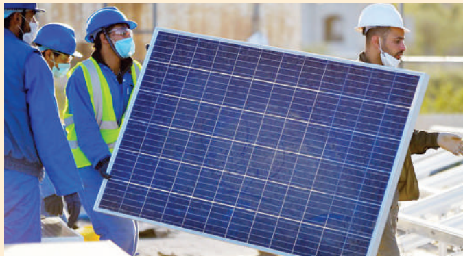
Workers install solar panels for a hospital in Yemen. (File photo)
