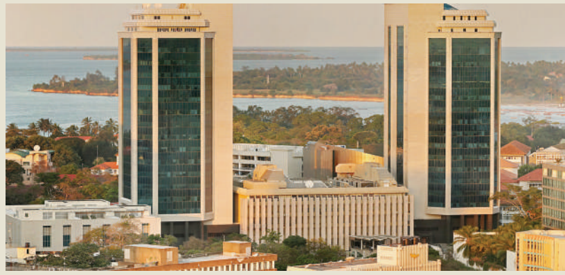
Bank of Tanzania headquarters in Dar es Salaam
