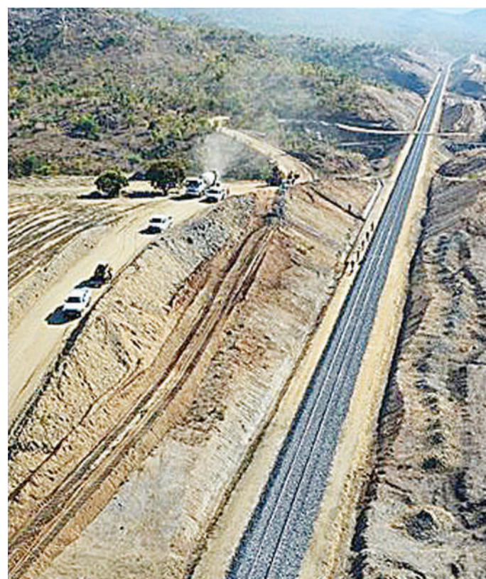
A construction site in Durban.
