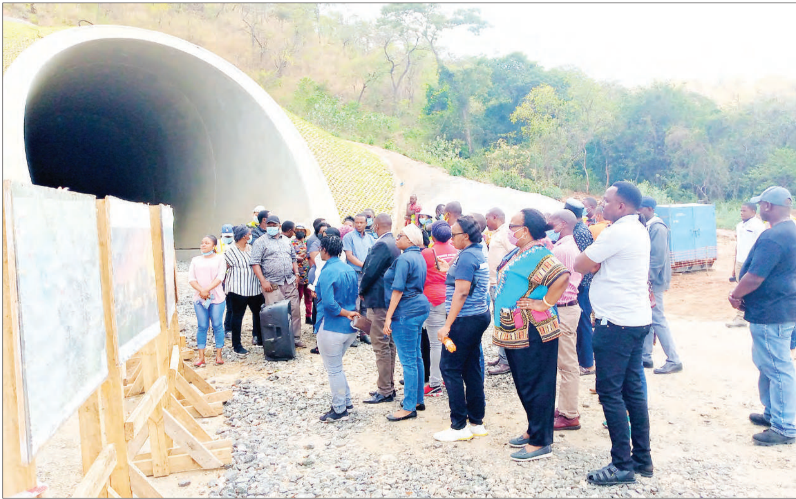
Staff from the Public Service Management and Good Governance wing of the President's Office view drawings of Standard Gauge Railways yesterday moments before being shown around a tunnel during their tour of the Kilosa District stretch of the Standard Gauge Railway, which is undergoing construction. Photo: Guardian Correspondent
