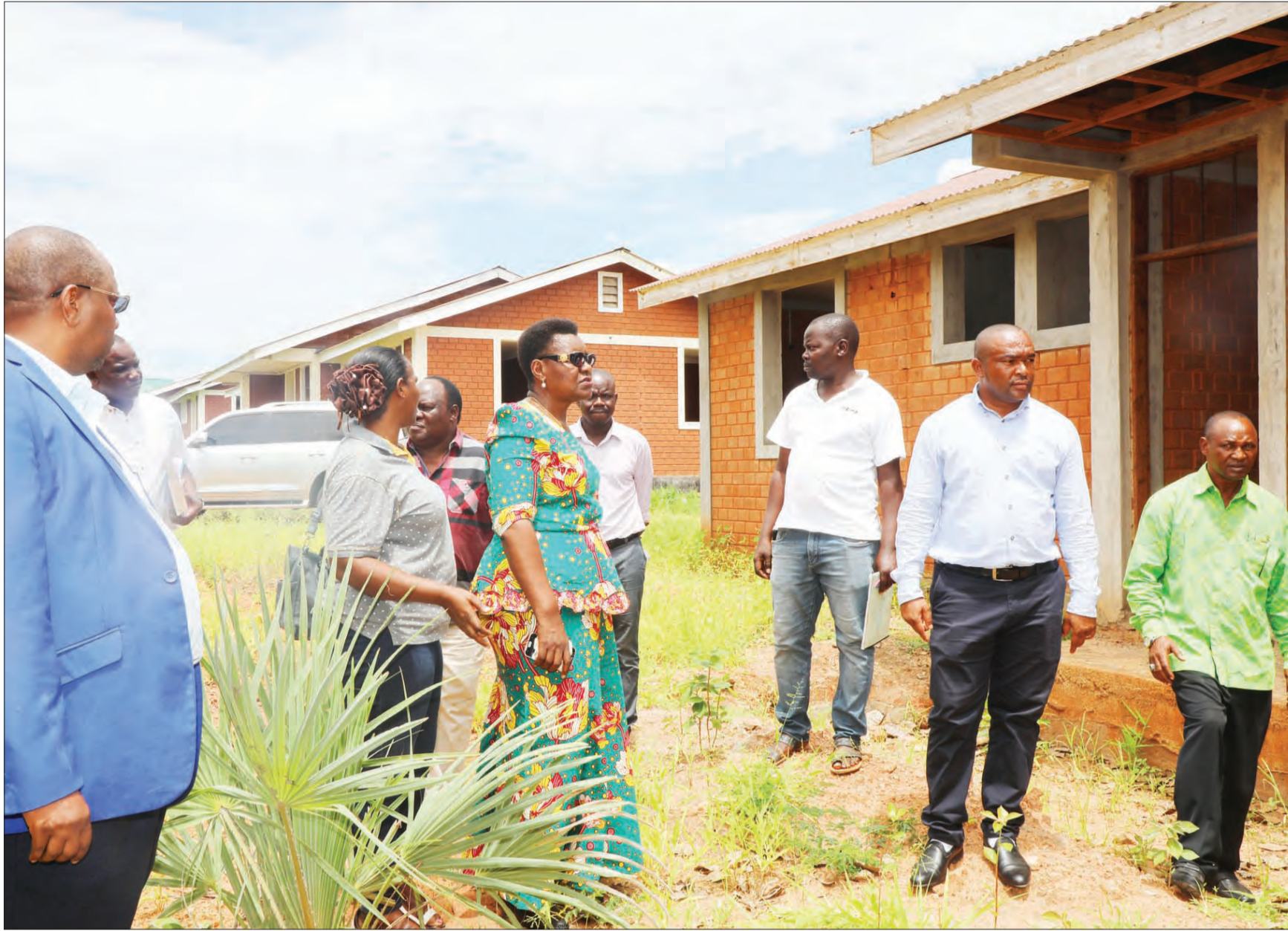
Deputy Minister for Land, Housing and Human Settlements Development Dr Angeline Mabula (C) inspects one of the National Housing Corporation (NHC) houses in Masasi district, Mtwara region yesterday. Left is the firm's communications manager Muungano Saguya. Photo: Correspondent Munir Shemweta
