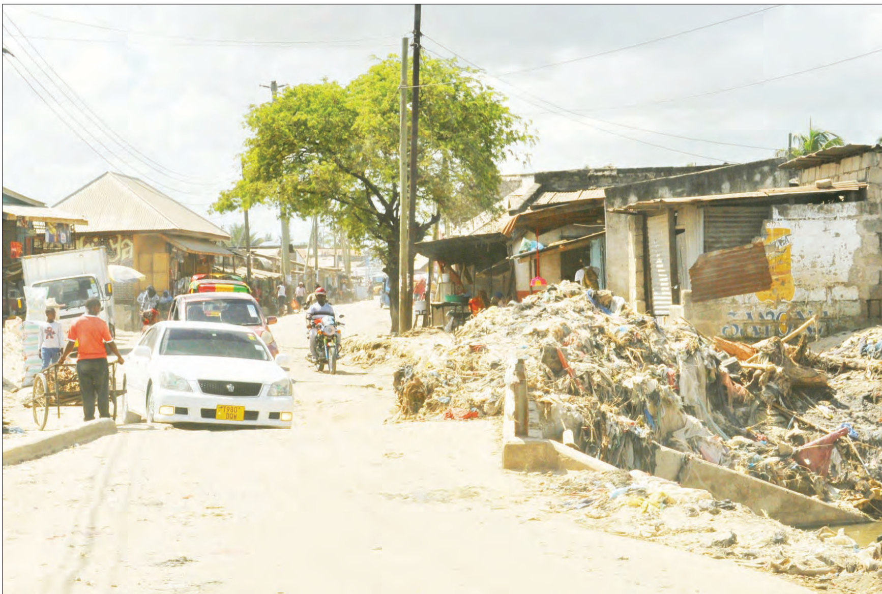
Vehicles drivers negotiate their way through a large pothole at Ng'ombe river bridge which links Kijitonyama Ali Maua and Tandale kwa Mtogole and also debris carried by flood in the outskirts of Dar es Salaam yesterday. Photo: John Badi
