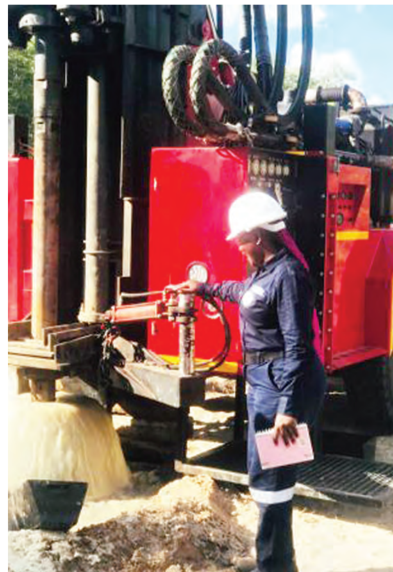
Alina Kadhila, a hydrogeologist at Namibia Water Corporation, operating a mud rotary drilling rig.
