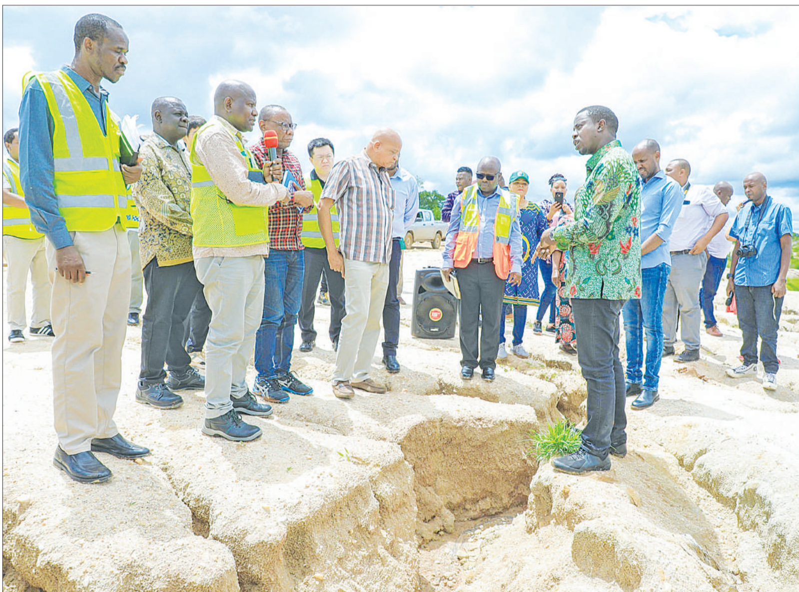
Works minister Innocent Bashungwa (R, nearest camera) gives instructions to Tanzania National Roads Agency (Tanroads) project manager Julius Msofe (with microphone) after inspecting the 120.8km Mkange-Tungamaa-Pangani road in Pangani District, Tanga Region, yesterday. Photo: Guardian Correspondent
