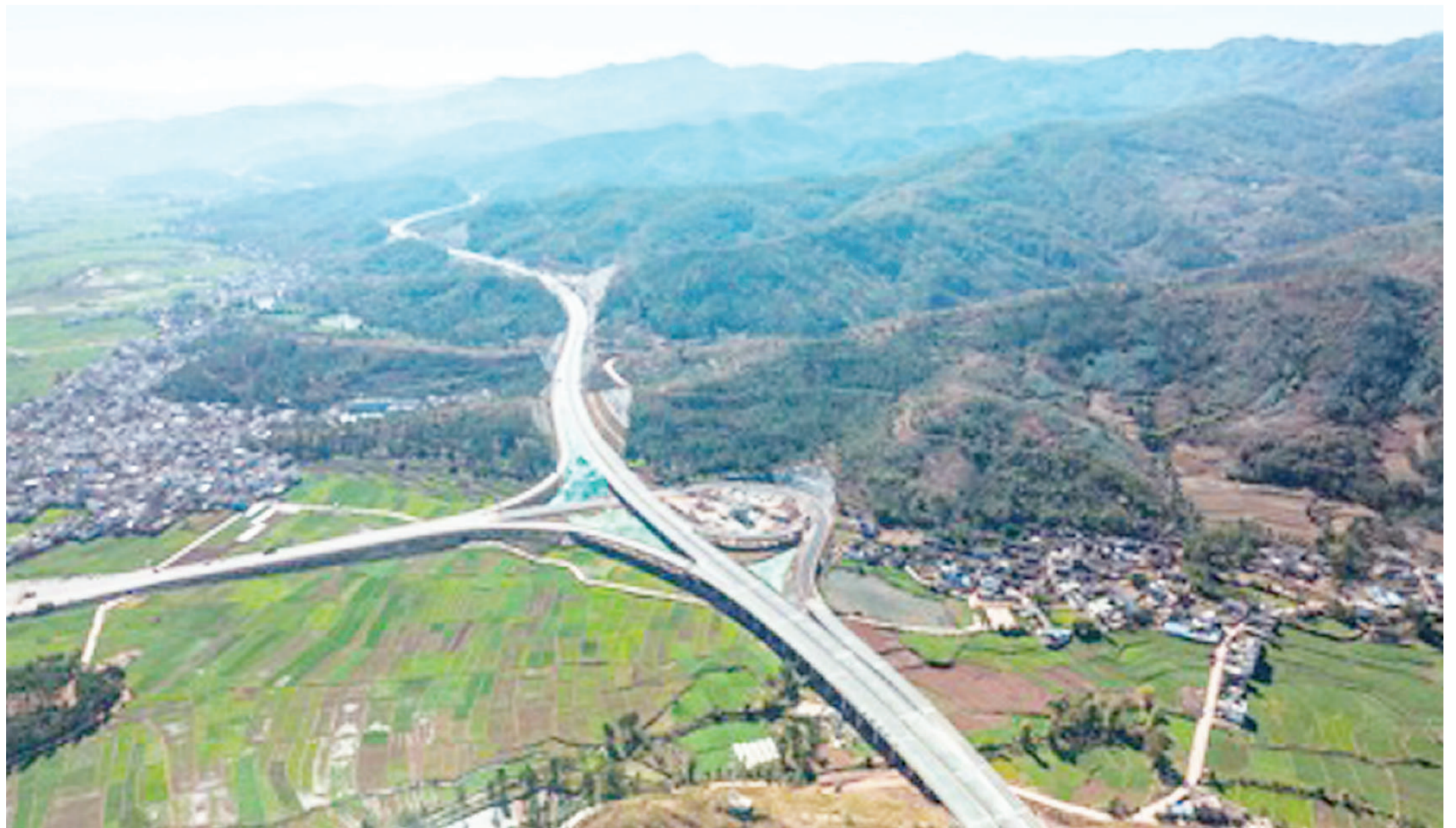
Photo taken on Dec. 16, 2021 shows a section of an expressway in Weishan county, southwest China's Yunnan province. File photo
