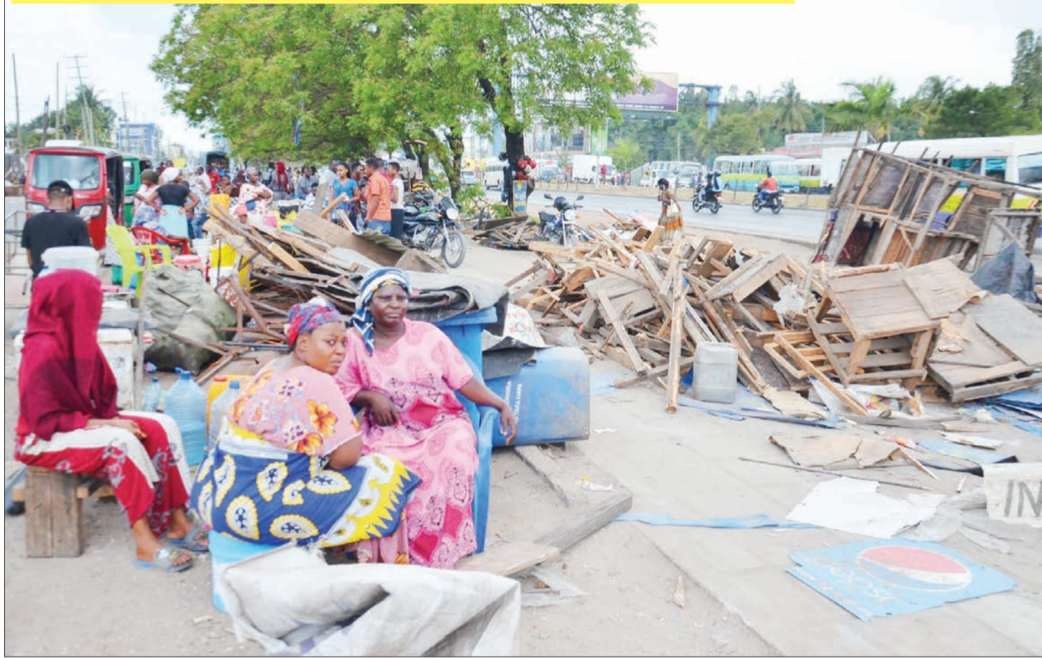
Food vendors assembled at a point in Dar es Salaam's Vingunguti suburb look on forlornly from the debris of stalls where they were based until Wednesday evening. That was only hours before tragedy struck - with a midnight demolition operation by the city militia. Photo: Correspondent Jumanne Juma
