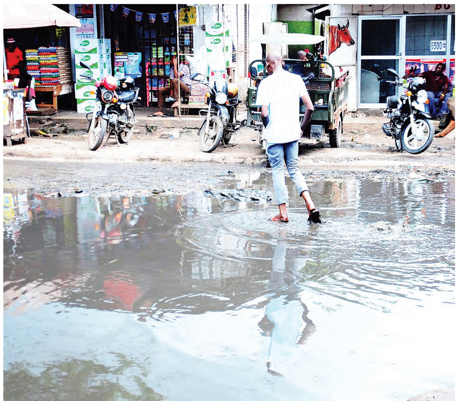
City resident walks in flood water which is dangerous, disgusting and dirty. It is a hazard to one's health, safety, and it could be deadly as captured at Buguruni market in Dar es Salaam yesterday. Photo: Correspondent Jumanne Juma
