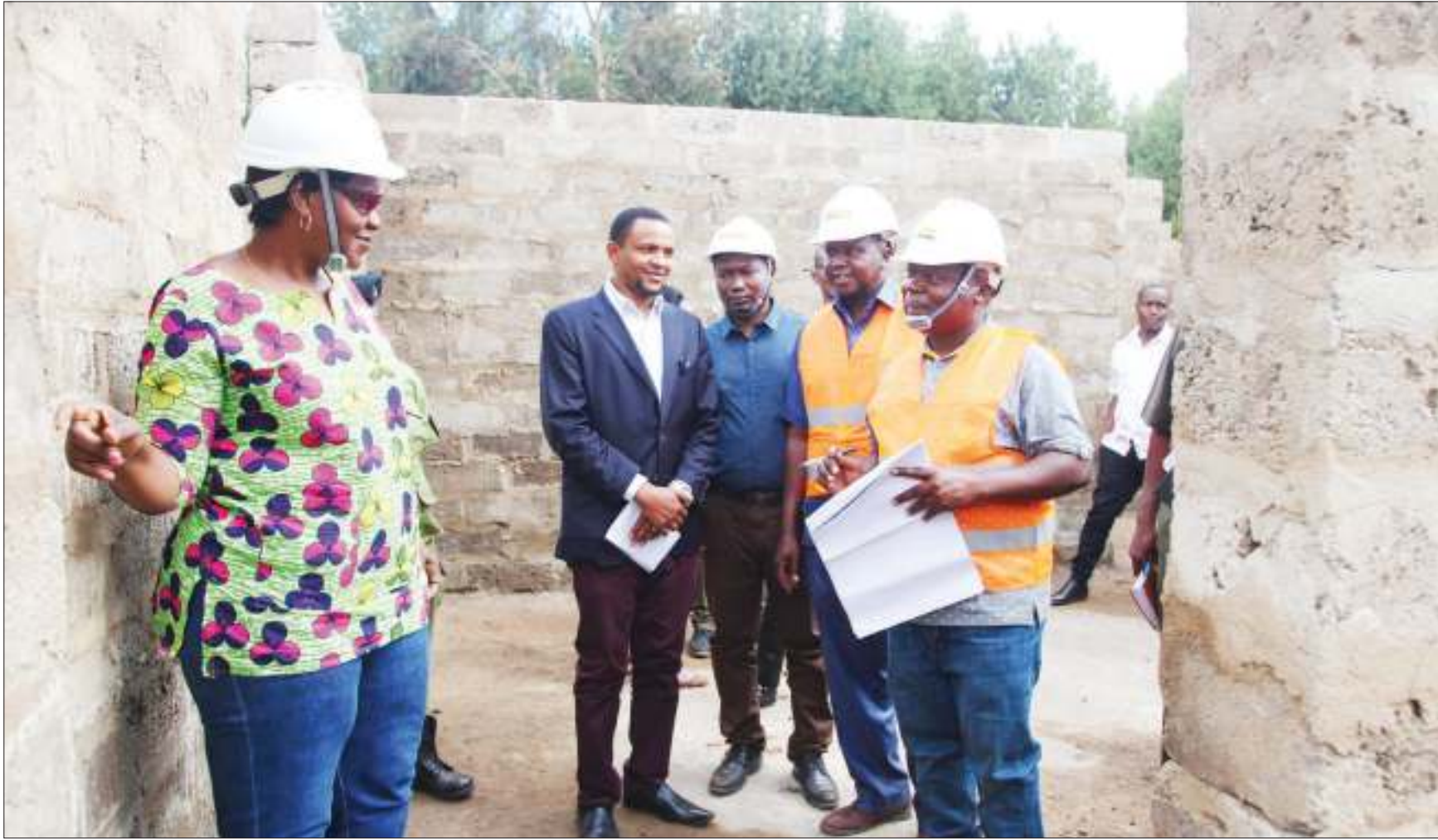
Lands, Housing and Urban Settlements Development Deputy minister Angeline Mabula (L) inspects the construction of Tanzania Forest Services offices at Rongai in Rombo district, Kilimanjaro region yesterday. Photo: Munir Shemweta
