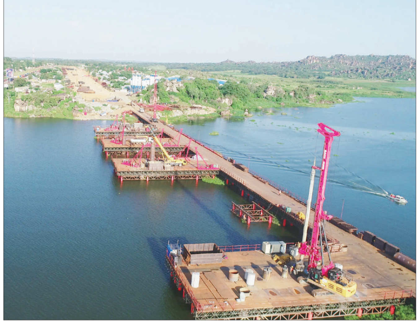
This is a temporary bridge built to facilitate the movement of materials for the construction of a 3.2-km-long permanent one across Lake Victoria waters - at Kigongo-Busisi in Mwanza Region - which is expected to cost 700bn/-. The scene was captured yesterday. Photo: State House
