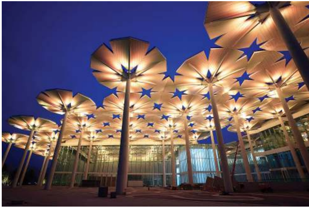
Photo shows a night view of the International Pavilion at the site of the International Horticultural Exhibition 2019 Beijing China (Expo 2019 Beijing) in Yanqing District of Beijing. (Xinhua)
