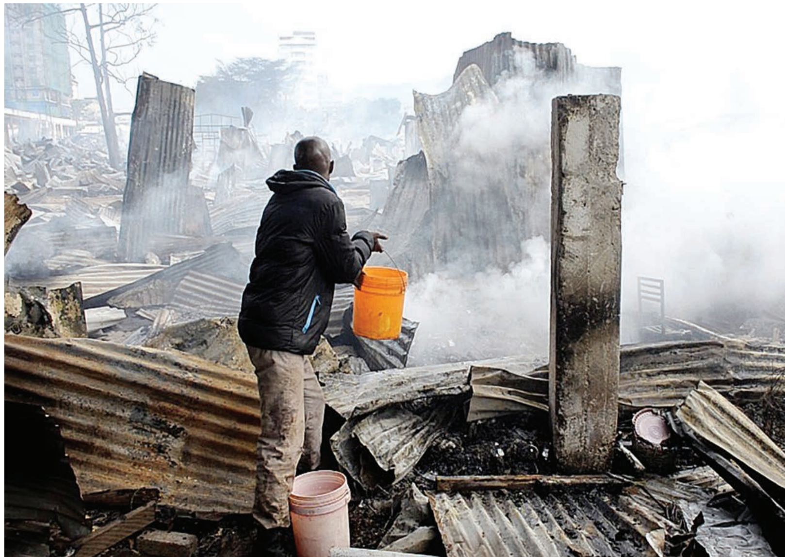
A trader moves to extinguish a fire at Samunge market in Arusha city yesterday, but long after it had inflicted extensive damage to goods and various other property. Photo: Correspondent Cynthia Mwilolezi
