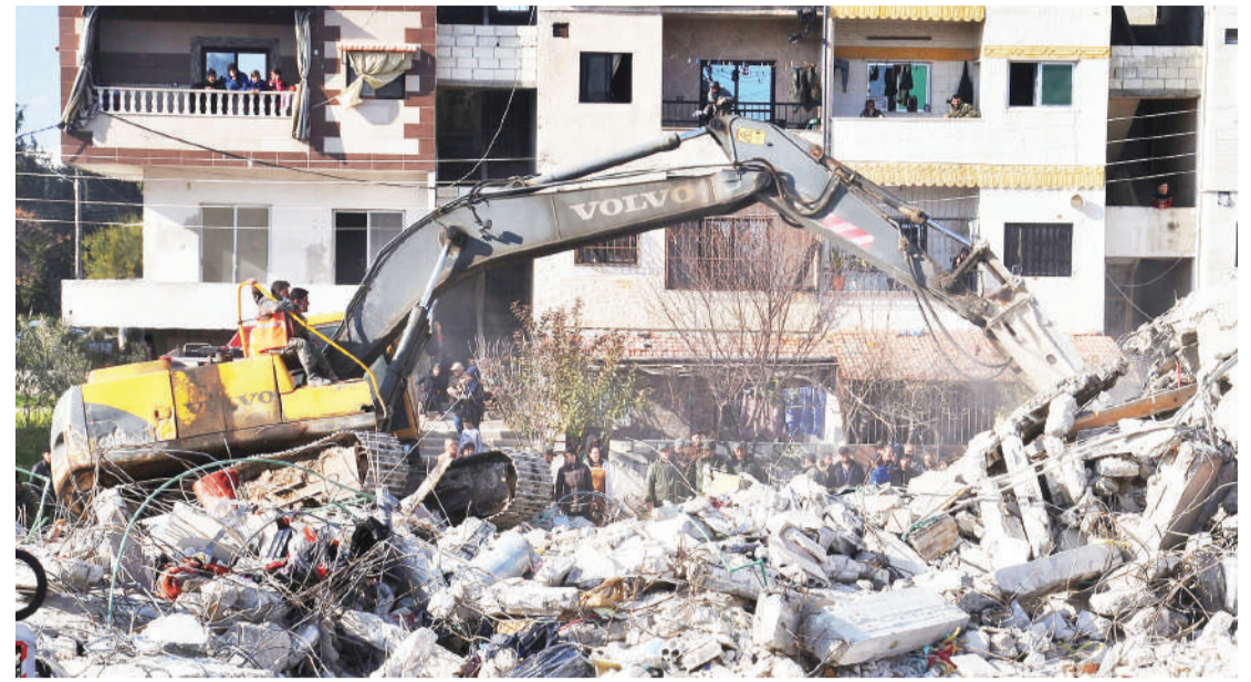
Rescuers work at an earthquake-hit site in Latakia, Syria, Feb. 10, 2023. (Str/Xinhua)
