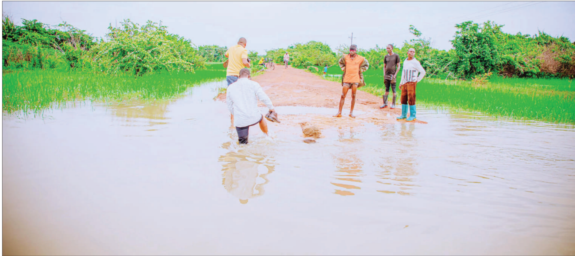
NO WAY THROUGH: Residents of Kisai village in Urambo District, Tabora Region, have no option but to wade through floodwaters yesterday as others look on helplessly - with heavy rains having rendered the strategic road pictured impassable. Photo: Guardian Correspondent
