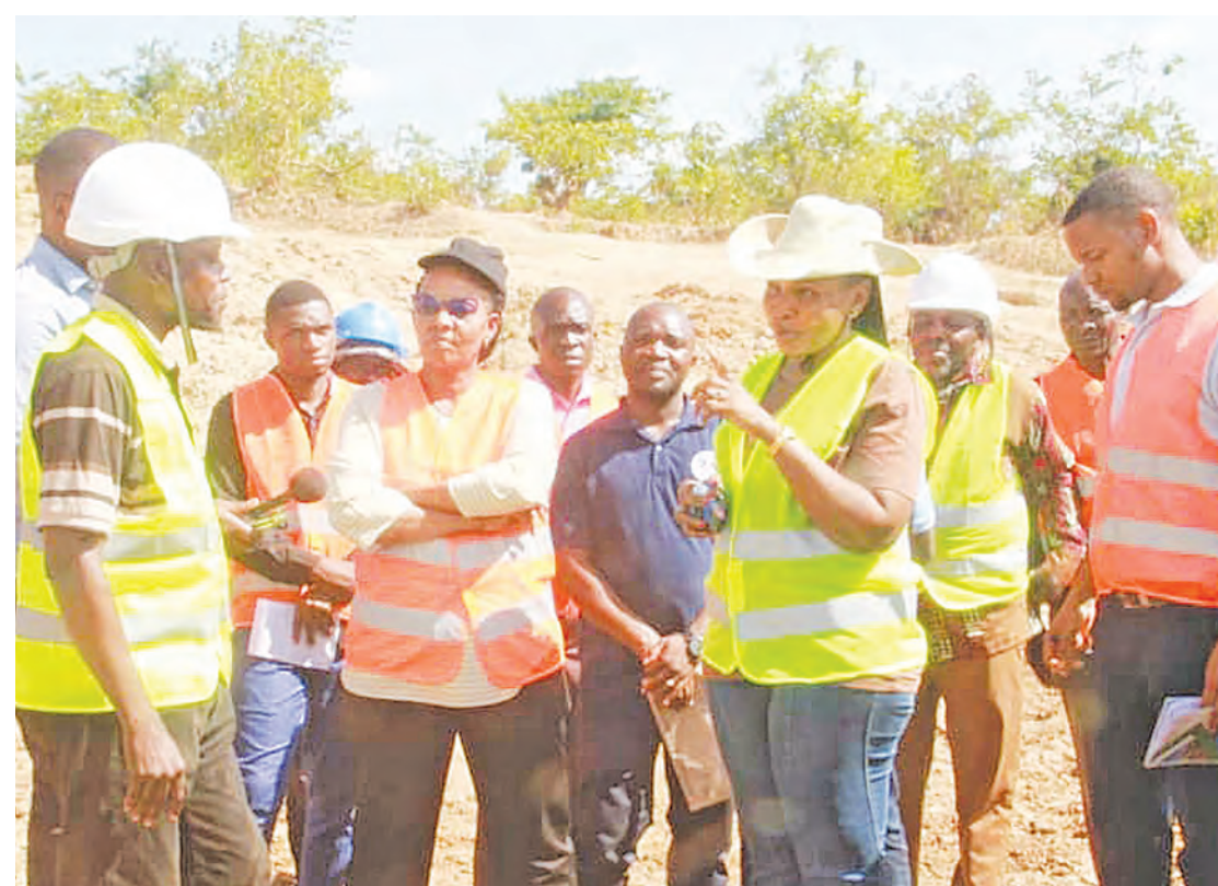
Songwe regional administrative secretary Happiness Seneda (3rd-R, gesturing) seeks explanation at the weekend from Janta Construction Co. Limited contractors in connection with obstructing the flow of water distributed under the Msangano-Naming'ong'o project. Photo: Correspondent Yasin Ibrahim
