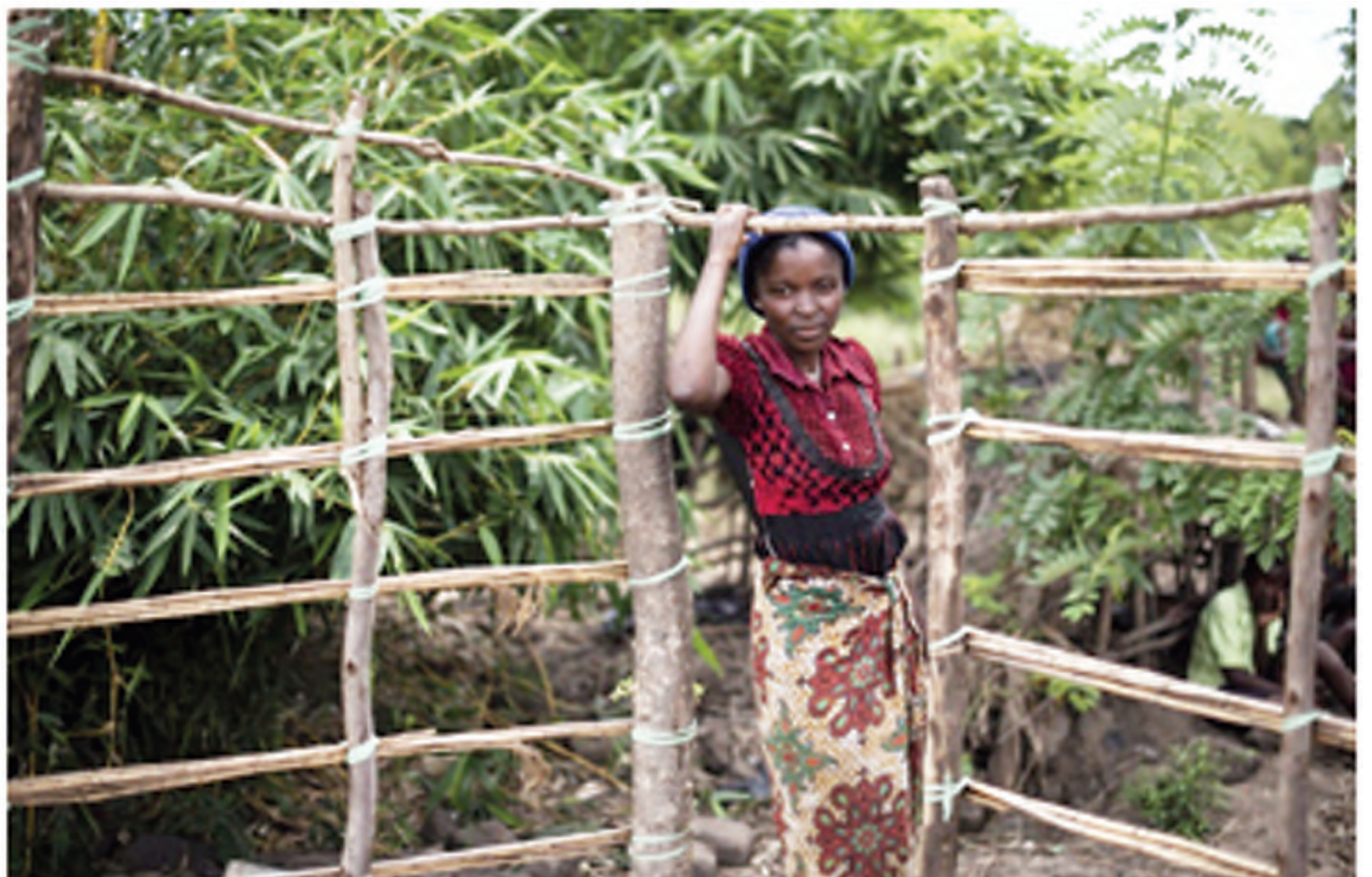
Dorothy, 27, stands inside the house she is rebuilding with her brother, in the village of Malambwe, southern Malawi, following the flooding brought on by Cyclone Idai. Dorothy's house collapsed and the floodwaters carrying away many of her belongings, as well as some of her livestock. She took her four-year-old child, and went to higher ground to escape the floodwaters. Credit: Philip Hatcher-Moore/Oxfam
