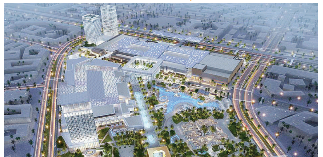
A bird's eye view of "KEC Hub" complex in Madinah.
