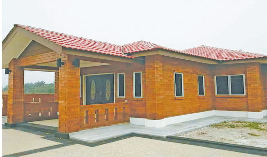
A house built using interlocking brick system. File Photo
