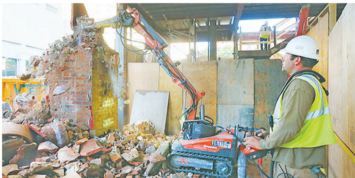
A construction worker uses controller for robotic arm on jobsite
