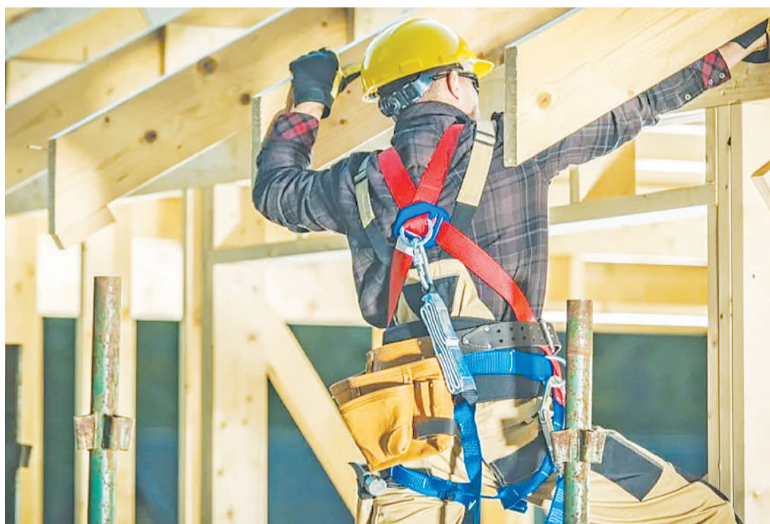
Construction worker working on single-family home. File Photo
