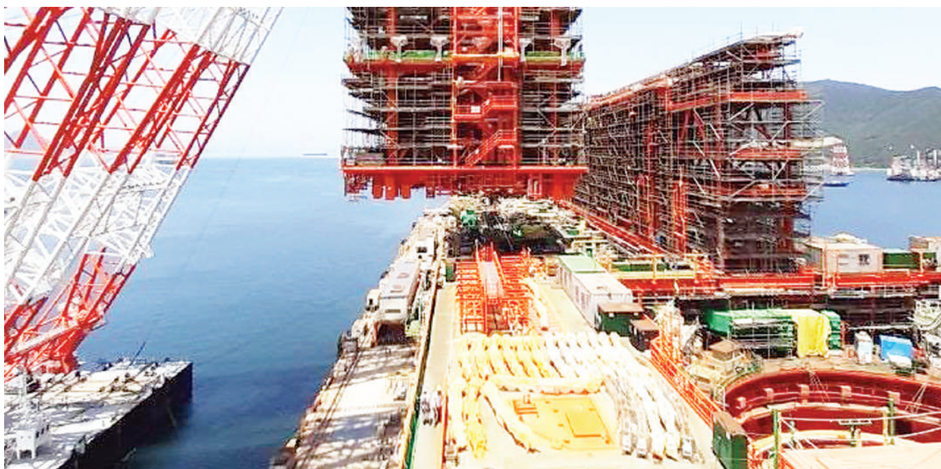
Assembling the Coral South FLNG plant in South Korea.
