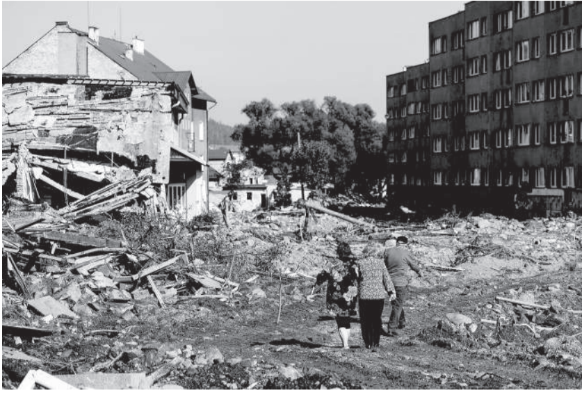
Residents walk in front of a building destroyed as a result of the heavy flood in Stronie Slaskie, southern Poland, on September 18, 2024. AFP
