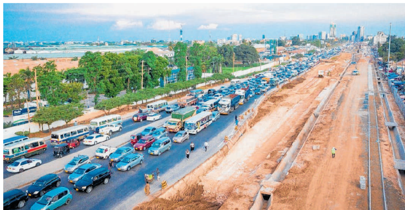
Ongoing Construction Work on New Bagamoyo Road
