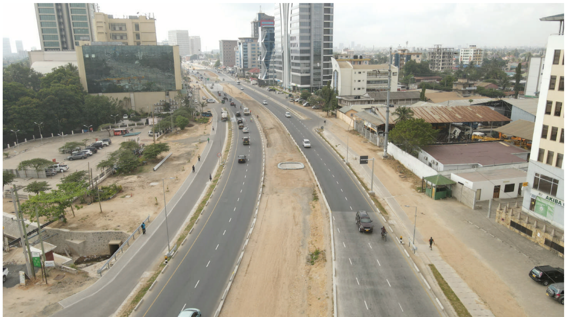
Completed new Bagamoyo road between Mwenge and Morocco intersections in Dar es Salaam.
