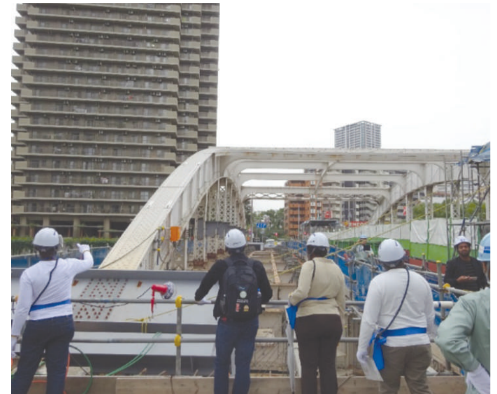
Visit to a Bridge Construction Site in Japan (Source: JICA)
