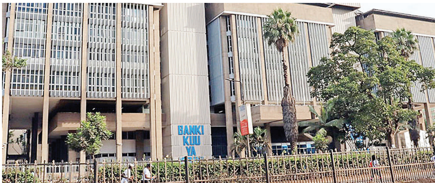
Central Bank of Kenya complex in Nairobi. File Photo.
