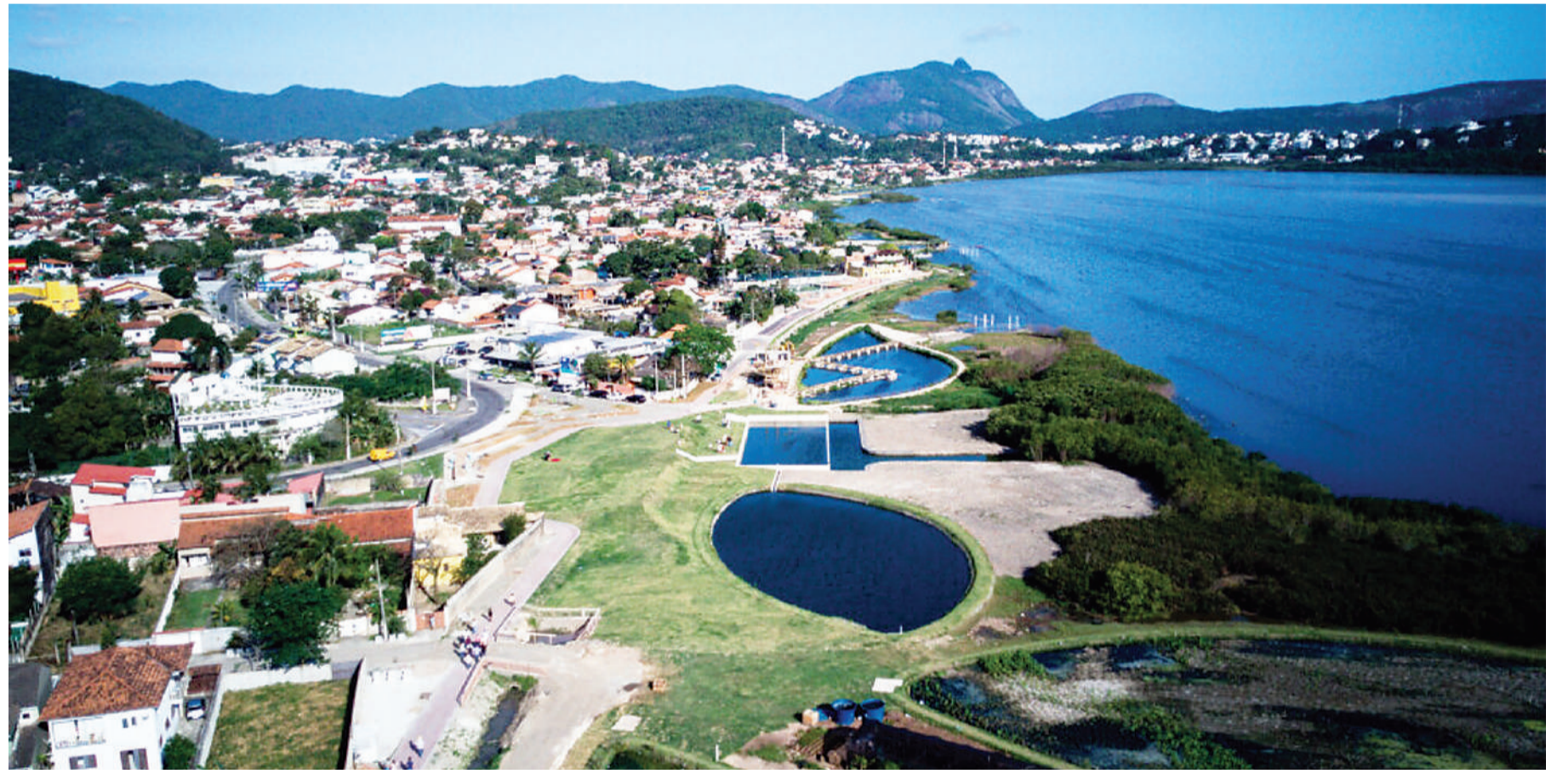
An aerial view of Hacienda Cafubá, on the north shore of Piratininga, a lagoon in southeastern Brazil, when ponds that serve as a spillway and to collect sedimentation of polluted water were being built and filter gardens that clean the water of the Cafubá River before discharging its waters into the lagoon were being planted. CREDIT: Alex Ramos / Niterói City Government
