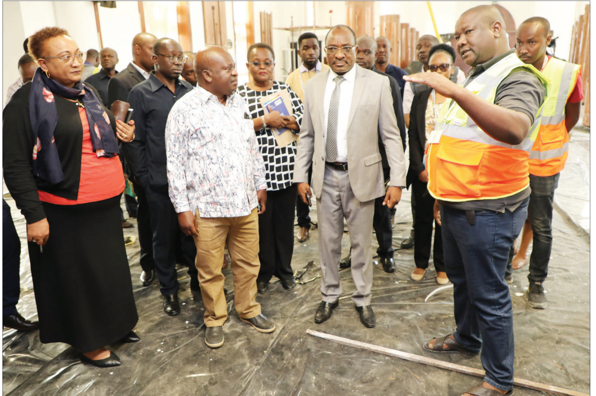
SUMA-JKT project engineer Bavid Pallangyo (R) briefs National Assembly Speaker Job Ndugai (2nd-L, foreground), who was assessing the ongoing rehabilitation of Parliament Building in Dodoma yesterday. Others are senior officials from the National Assembly, SUMA-JKT and the Tanzania Building Agency. Photo: National Assembly.
