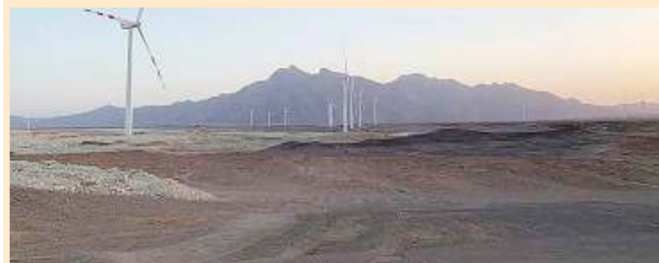
Ras Ghareb Wind Energy is the first wind farm tendered on BOO scheme and is part of the Egyptian government's drive to increase the share of renewables in the energy mix with a target wind generation capacity of 7 GW by 2022.
