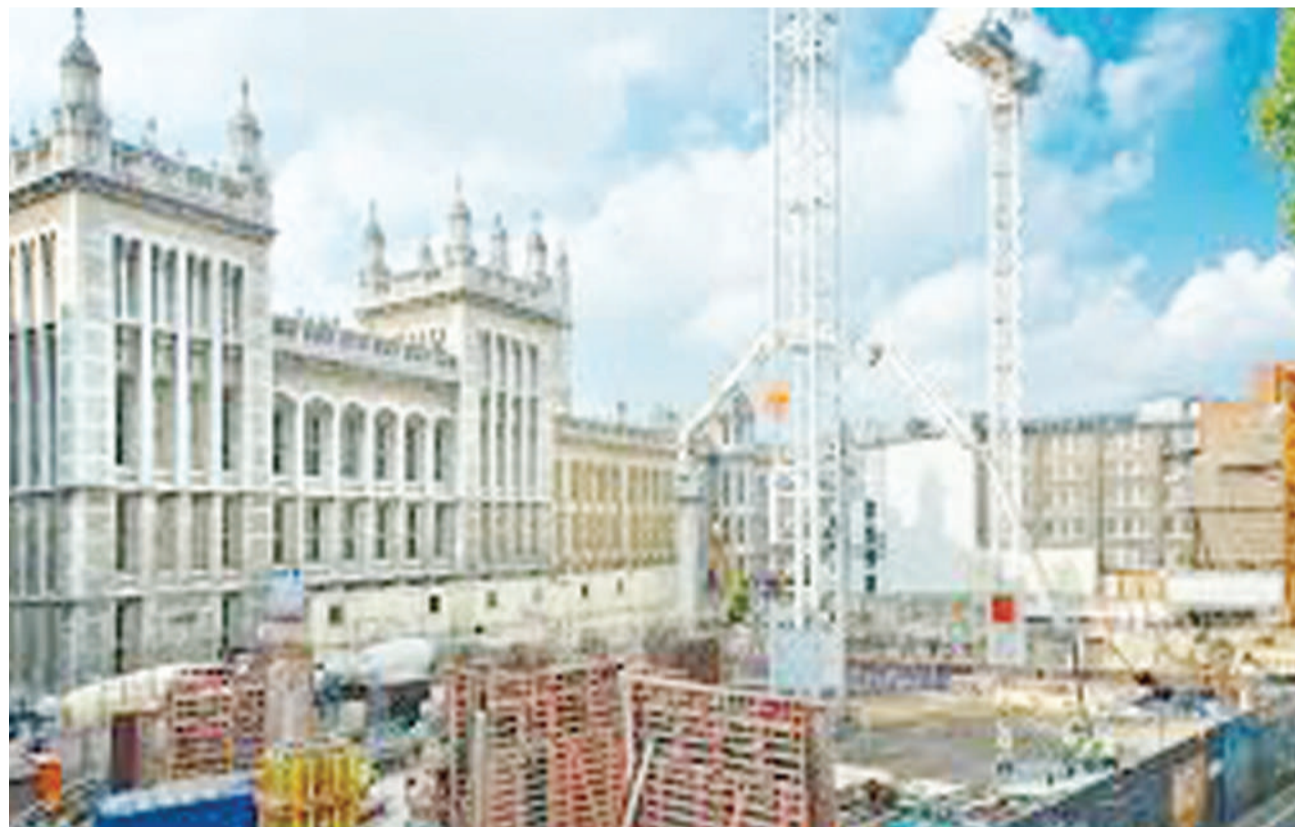
A construction site in London.
