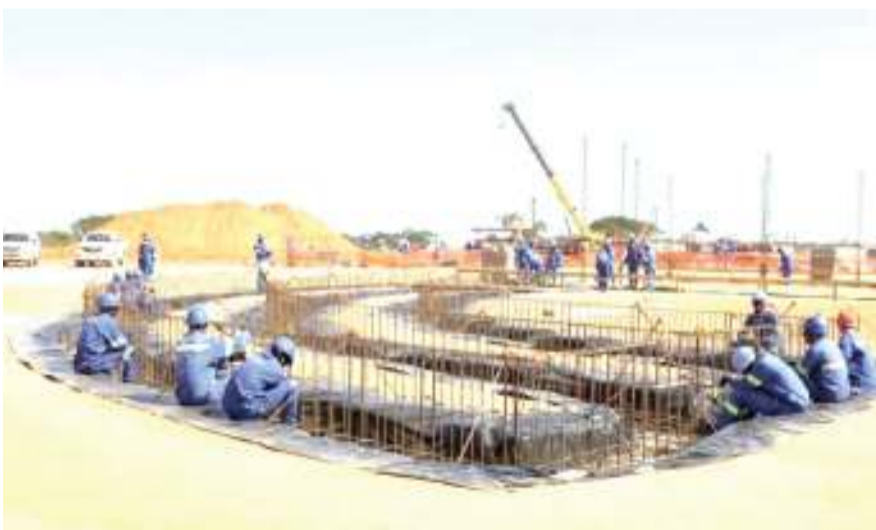
Construction work of Rovuma LNG plant going on in northern Mozambique.
