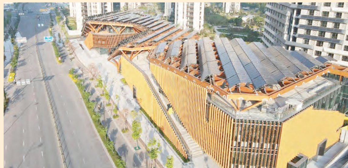
Photo shows a zero energy and zero emission community service center of a rental housing project for talents in Nanjing, east China's Jiangsu province. The building adopts a wooded structure and comes with a rooftop photovoltaic power generation system. (People's Daily Online/Wu Jun)
