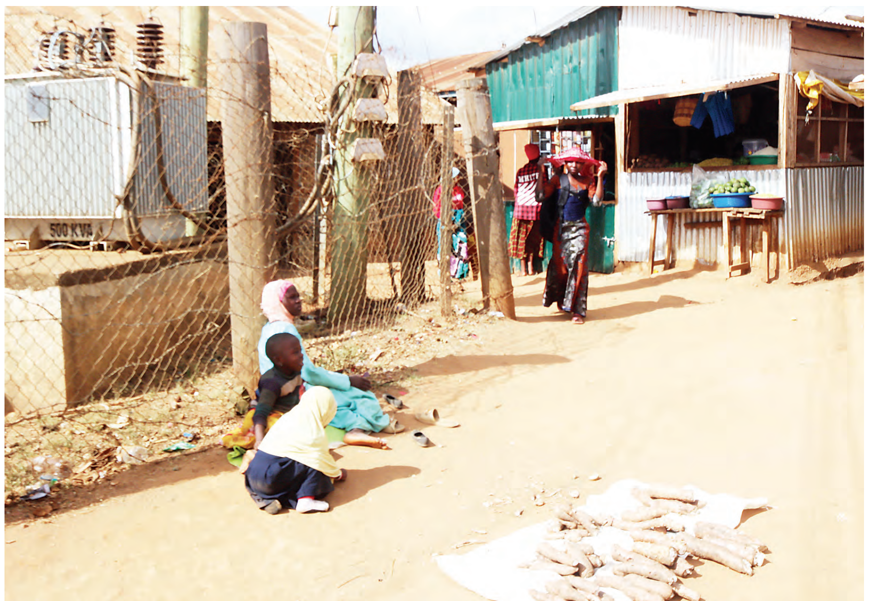
A small trader seated dangerously with her two young children near a high-voltage transformer at Songe market in Kilindi District, Tanga Region, at the weekend while waiting for customers for her cassava. Photo: Correspondent Dege Masoli
