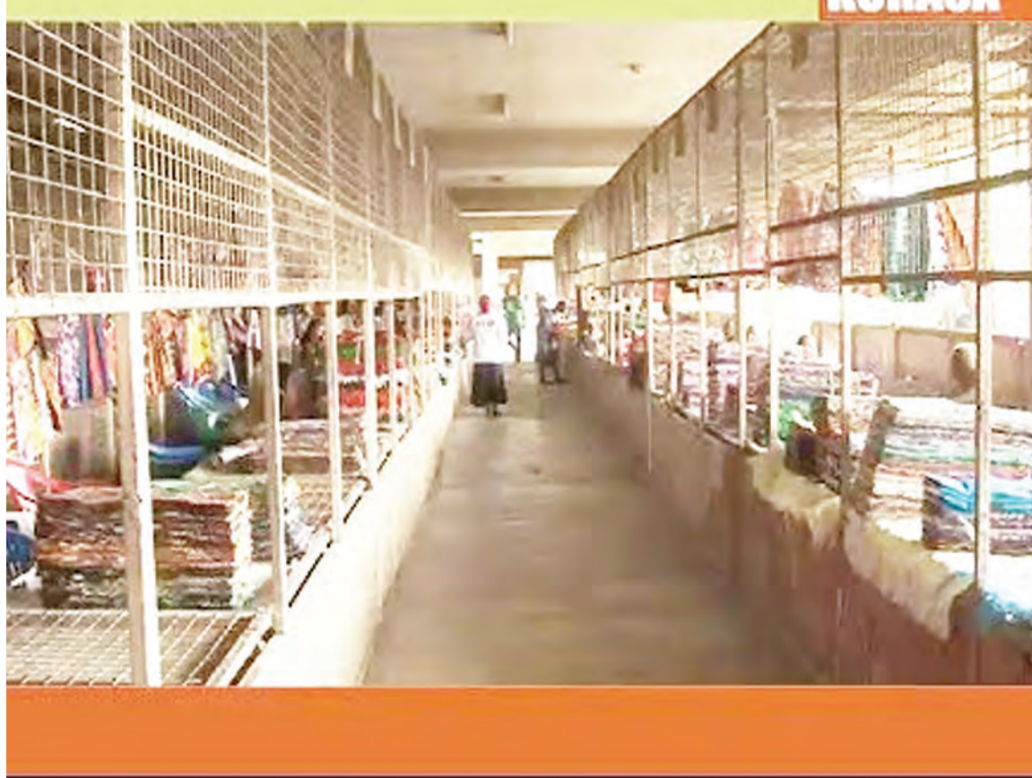
Could this building really offer a pleasant shopping experience? Originally designated to accommodate many thousands of traders, like the Machinga complex in Ilala, Dar es Salaam, had been rejected by sellers and customers alike. But who sanctioned the go ahead, and should bad decisions that incur huge losses for the nation be investigated?. File Photo
