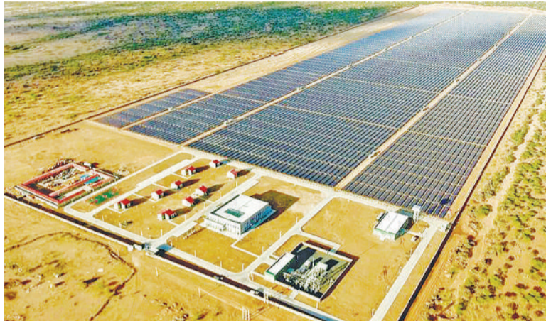
China-financed solar power plant in Garissa County, Kenya
