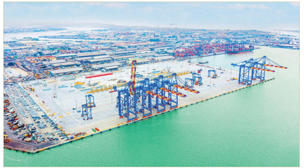
The expansion project of Abidjan Port in Cote d'Ivoire, built by a Chinese company, is a significant achievement of China-Africa cooperation under the framework of the Belt and Road Initiative. Since its inauguration in 2022, Abidjan Port has experienced a notable rise in its capacity, promoting local economic and social development. Currently, Abidjan Port has become a crucial hub in West Africa. Photo shows Abidjan Port. (Photo by Chuai Zhichao)
