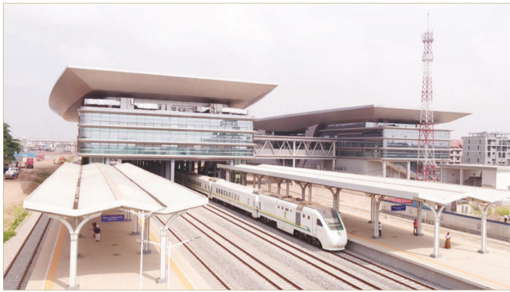
The Chinese-built Lagos-Ibadan Railway in Nigeria connects Nigeria's economic center Lagos and the south-west industrial city Ibadan, which not only facilitates people's travel, but also helps improve the efficiency of port and inland cargo transportation. Photo shows a train at a railway station along the Lagos-Ibadan Railway in Nigeria. (Photo by Lan Yuanhong)
