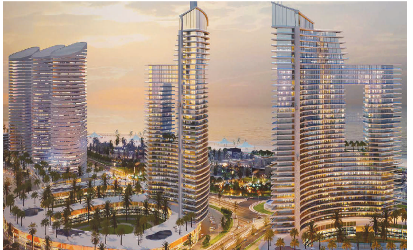
Marina Towers project in Egypt's New Alamein City.
