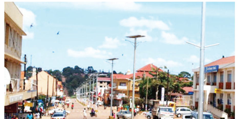
Solar lights installed along Edward Avenue in Masaka Town.
