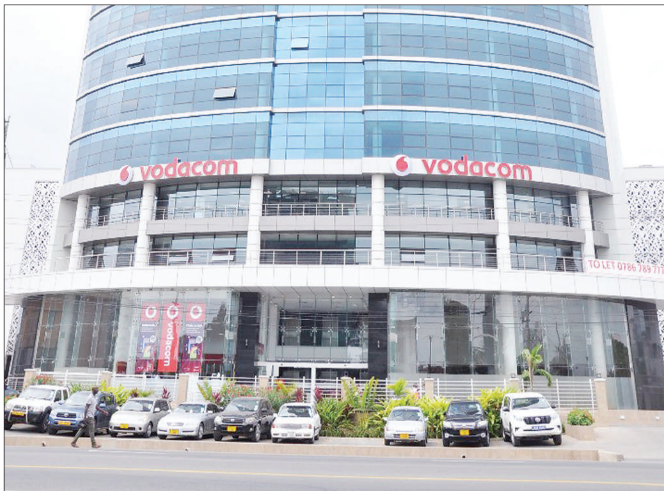
Vodacom Tanzania Plc's head office in Dar es Salaam.
